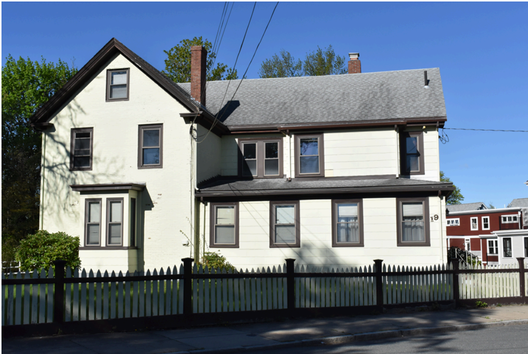
Figure 3. Daniel Withington House, east elevation, looking west from Ashland Street (The Public Archaeology Laboratory, Inc. 2021).
