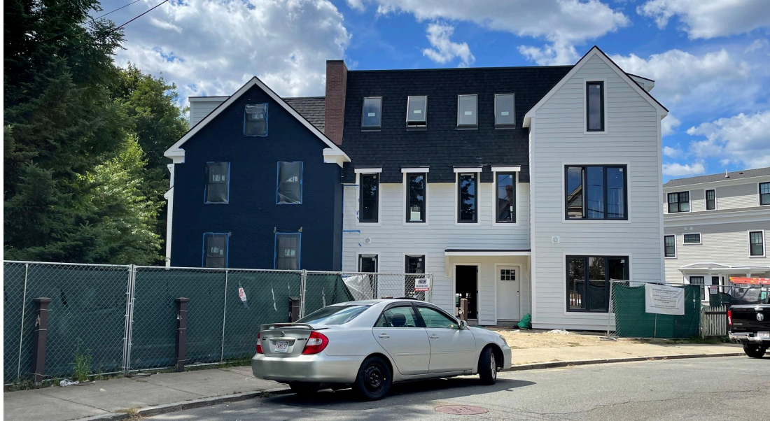
Figure 11. Daniel Withington House, east elevation, and new addition (Chelsea Blanchard, October 2024)
